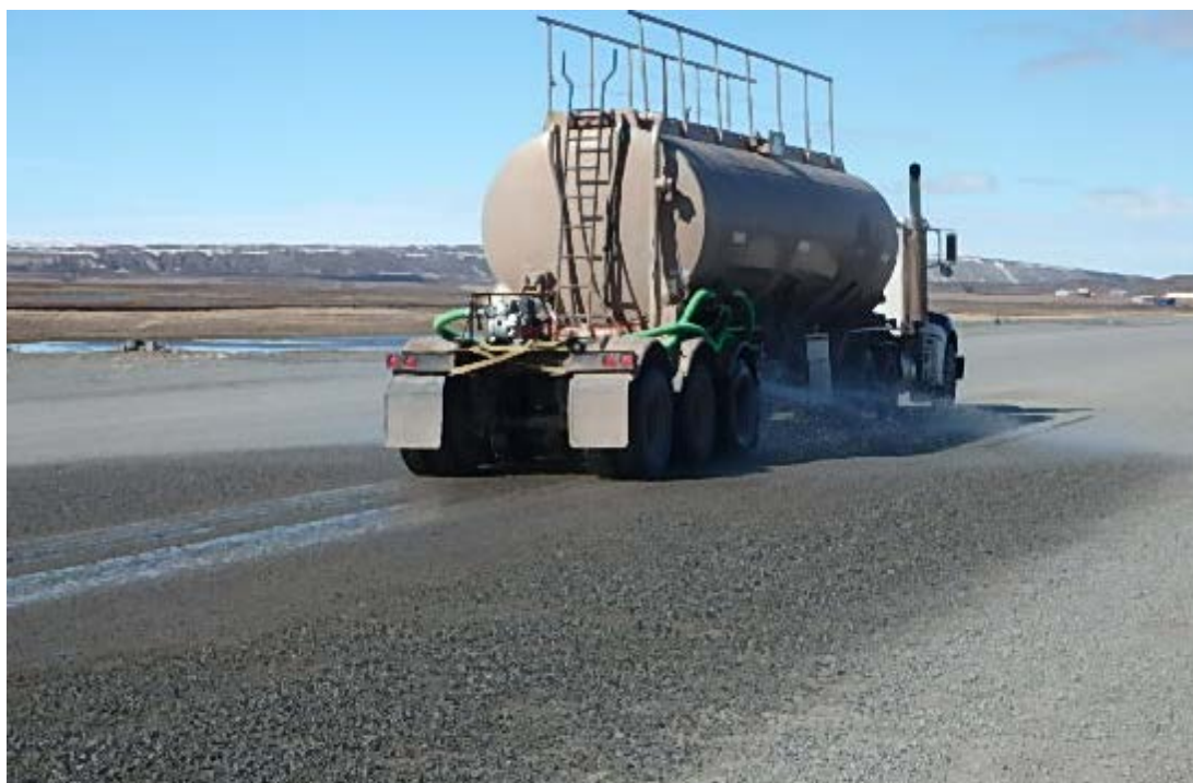
Figure 8 Application of water along the airstrip (provided by Baffinland, October 2025).
