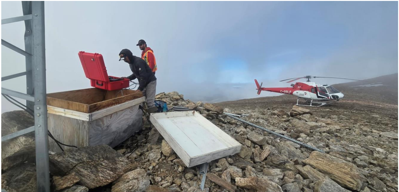
Figure 4.2 Helicopter Support for VHF Repeater Repairs
