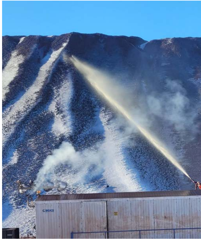
Photo 7-6. DusTreat application to the Milne Port ore stockpile, March 11, 2023.
