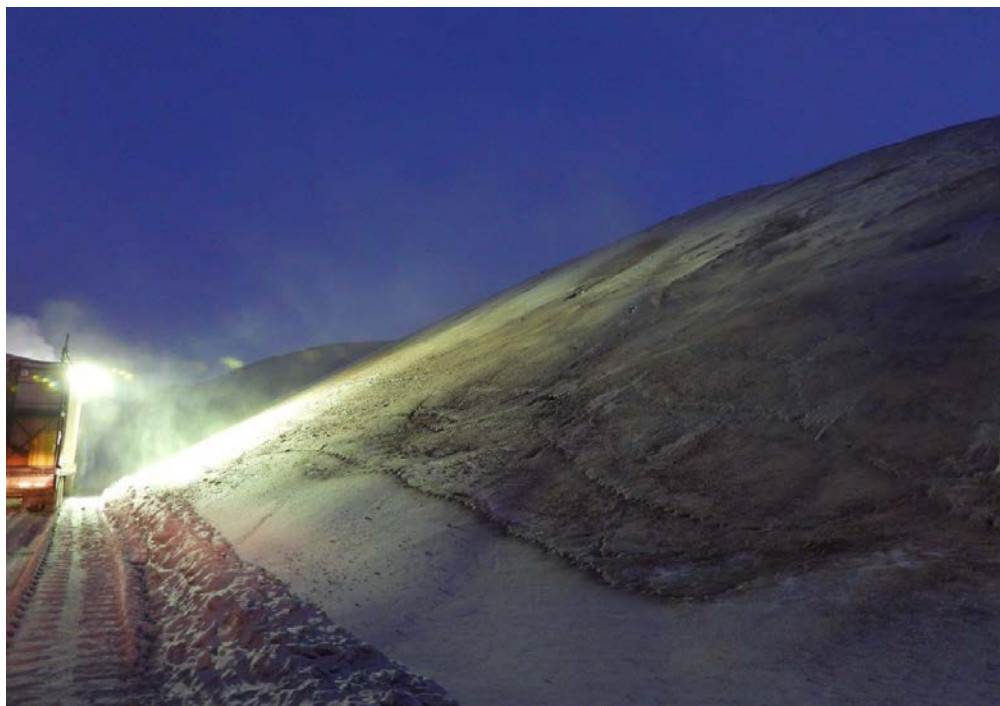
Photo 7-5. DusTreat application to the Milne Port ore stockpile, January 15, 2023.
