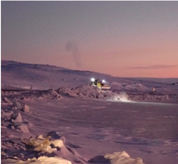
Photo 9-7. Snowbank management (in progress) to facilitate wildlife crossing and improve driver visibility.
