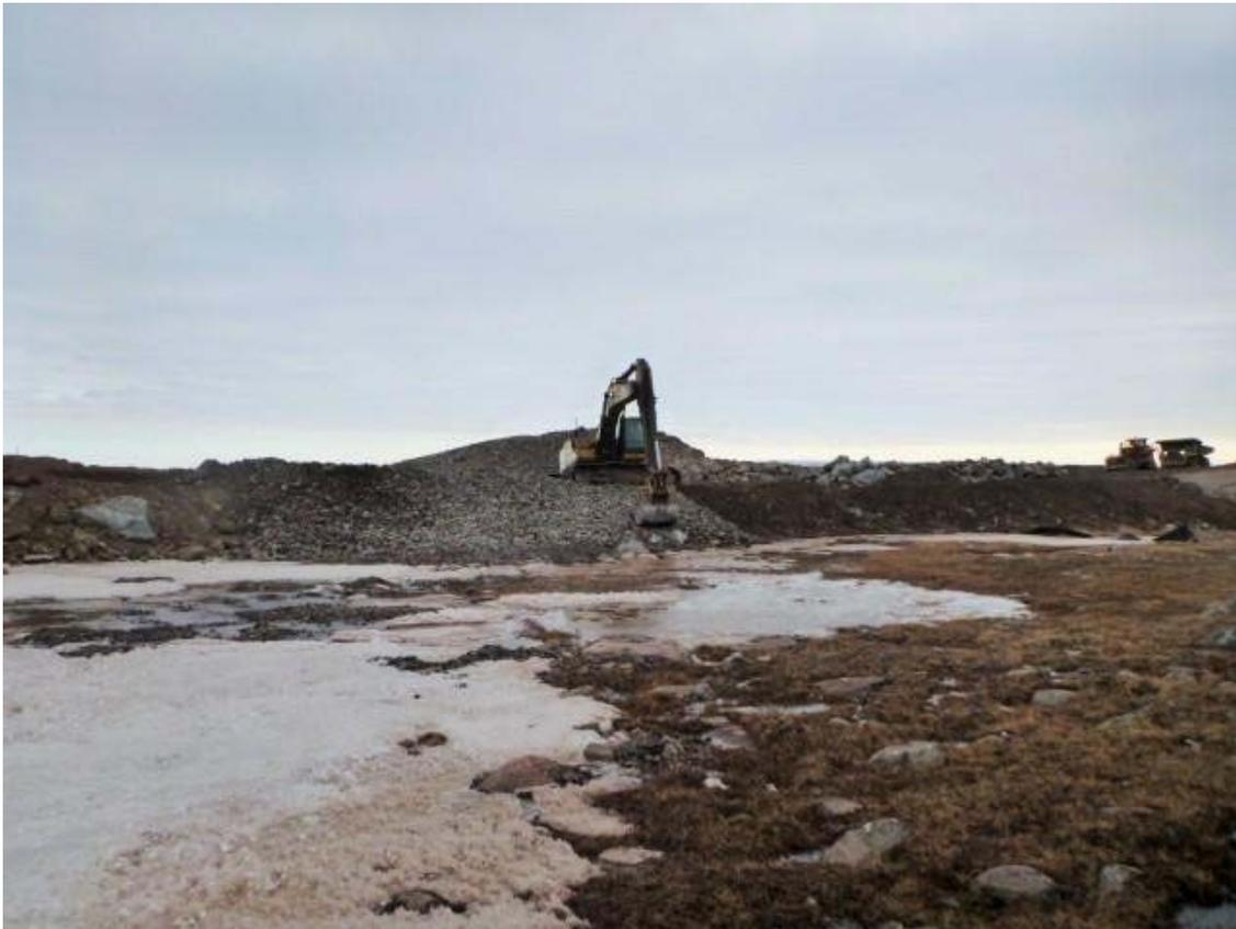
**Photo 21 - Excavator armoring the Mine Haul Road embankment, May 2016**
