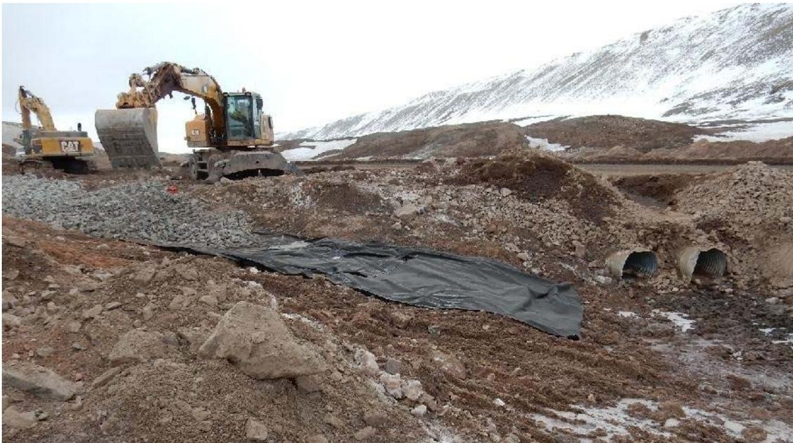
**Photo 22 - Milne Port Tote Road Km 90 ditch and culvert repair and armoring, June 2016**
