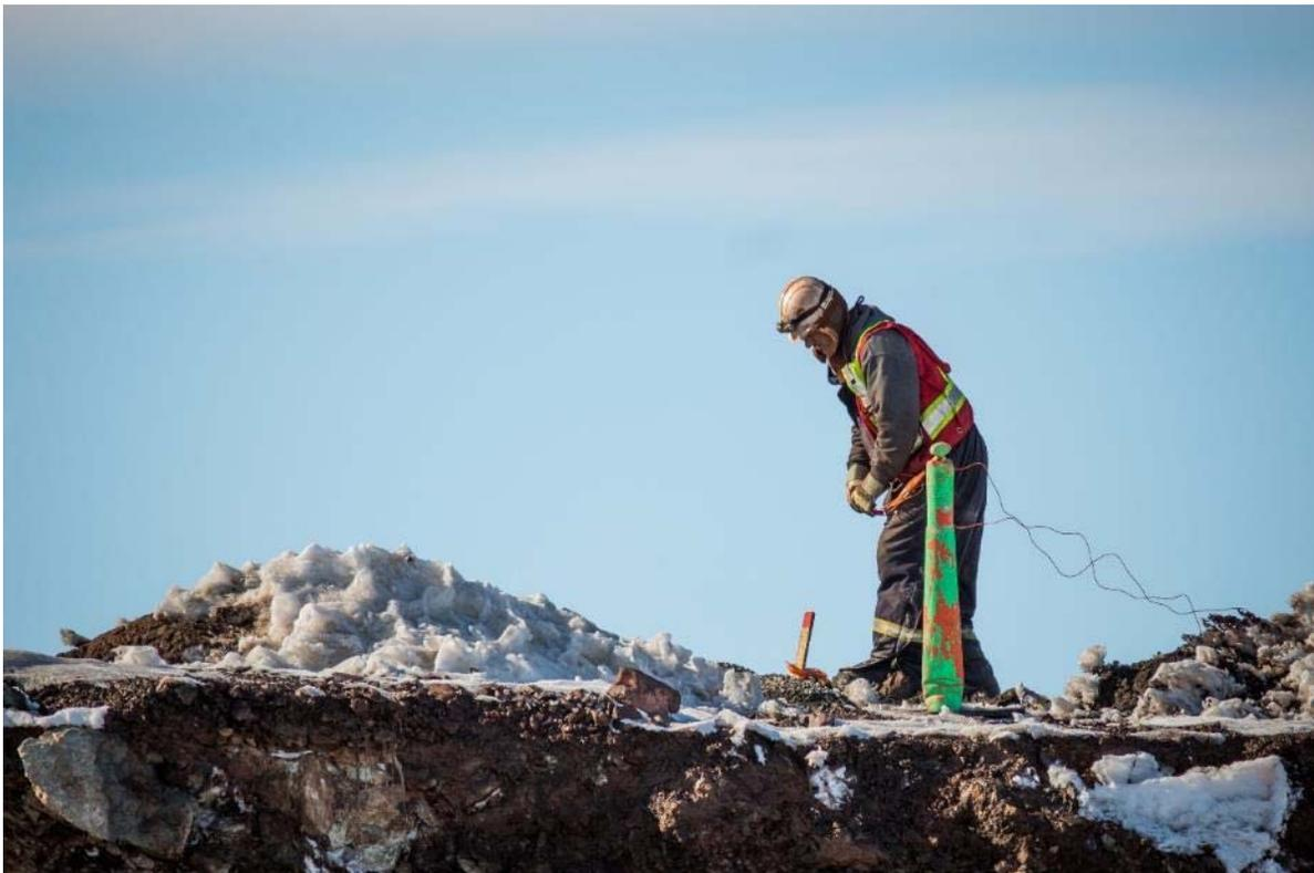
**Photo 2 - Prepping for blast at Deposit #1**
