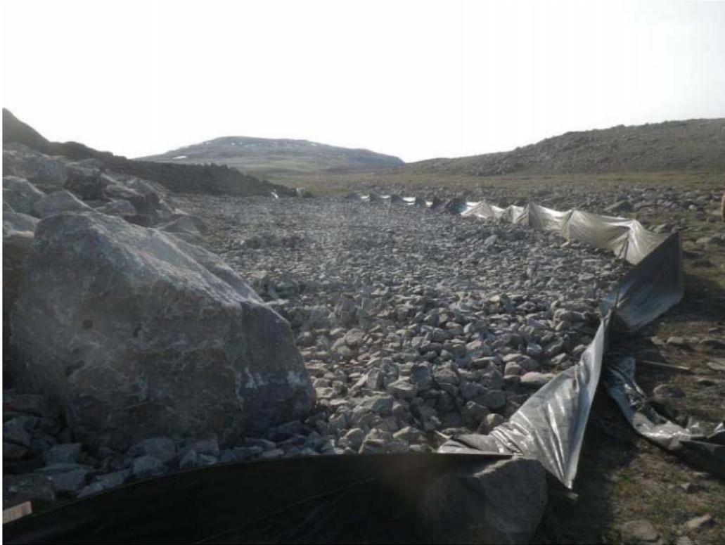
**Photo 23 - Siltation mitigation measures at the toe of the Crusher Pad, July 2016**
